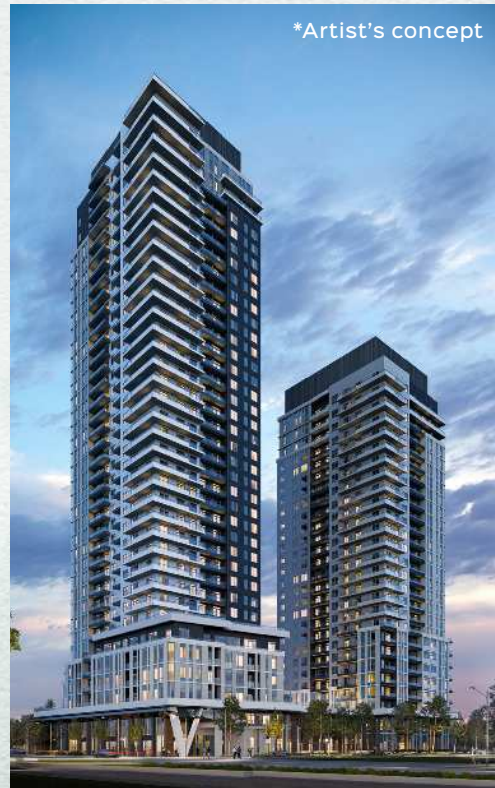
The Vincent VAUGHAN Under Construction
